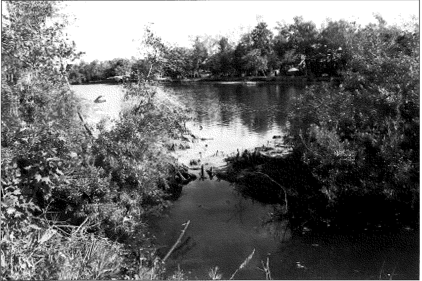
Figure 6. Northeasterly view of the breach. Steven Kingsley property in Sections 6 & 7, T-7-S, R-9-W, Harrison County, MS
